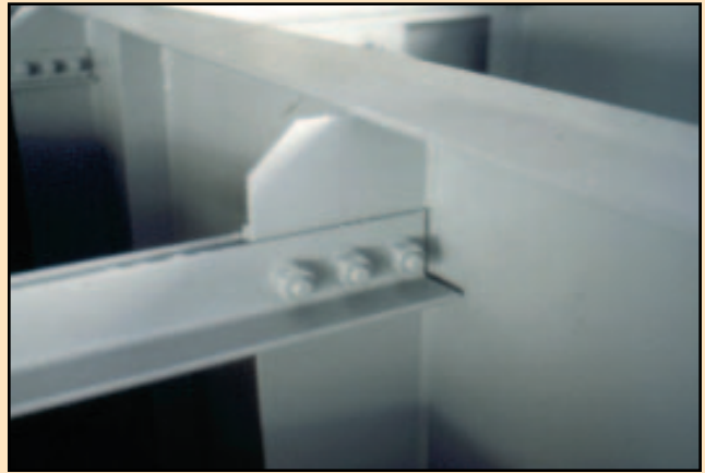
In-shop coating offers a number of application benefits, including better assurance of a uniform thickness, even in tight crevice areas.
