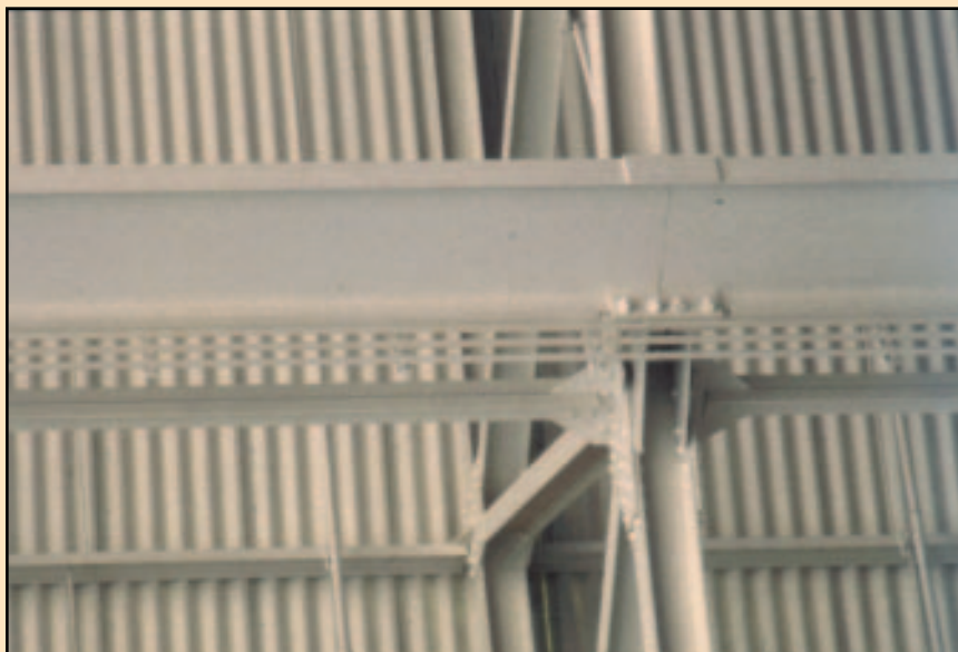
Significant cost savings can be realized by in-shop coating of structural steel, partly because enhanced application efficiency and the elimination of delays caused by adverse conditions.
