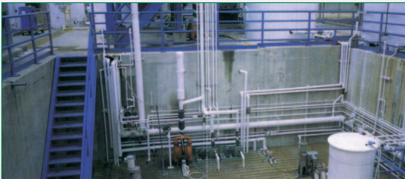
MSI has an award-winning, computer-controlled, multi-million-dollar waste treatment system that utilizes gravity flow from all process areas. (The lines from the new building are routed into the system.) The treatment area is housed outside the two plants in a 20-ft-deep concrete vault. The set-up allows easy access and quick, visual inspection of the stainless steel tanks.
