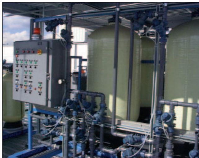
Kaynar has recently installed a new rinsewater treatment system. To the right of the control panel are the DI resin units. The smaller resin columns visible to the left are for the cyanide treatment system.
