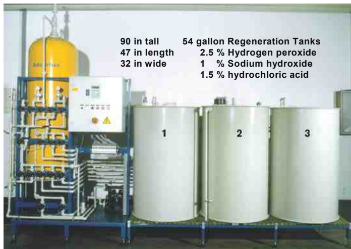
Figure 7, Design of an Adsorber Polymer Unit with its three regeneration tanks
