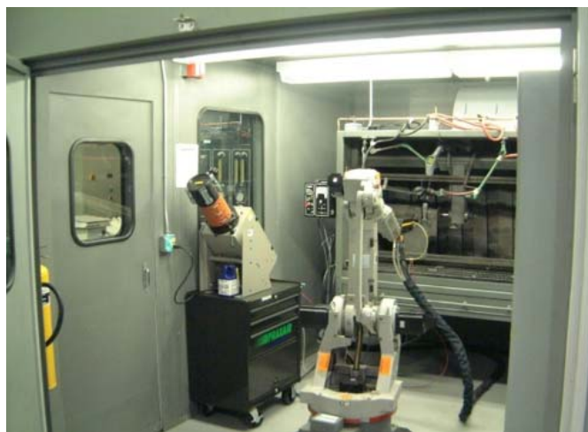
Figure 3. Inside of HVOF Spray Booth at OO-ALC.
