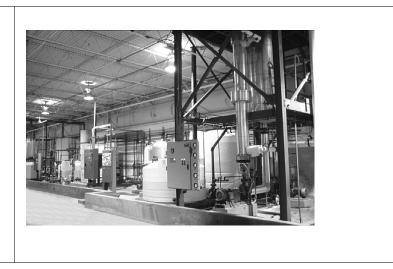
By using the DPU system, the cost of operation is reduced to the point where recovery becomes economical for any plant consuming more than two truckloads per month of 80% acid. Several installations have been installed over the last fifteen years and, in all cases, acid recovery efficiencies in excess of 85% have been reported.
