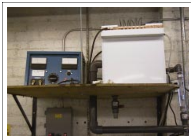
Figure 1. Electrowinning Rectifier and Electrolytic Cell
