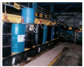
Drums in the chemical feeding station are clearly marked and safely diked for containment.
