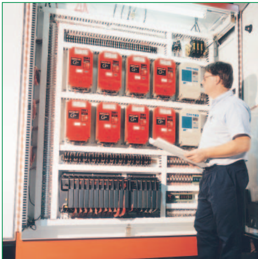
Jim Panzer, Krueger's control engineer, checks the central control panel housing the PLC and other equipment. The panel is located next to the operator control book for easy access.
