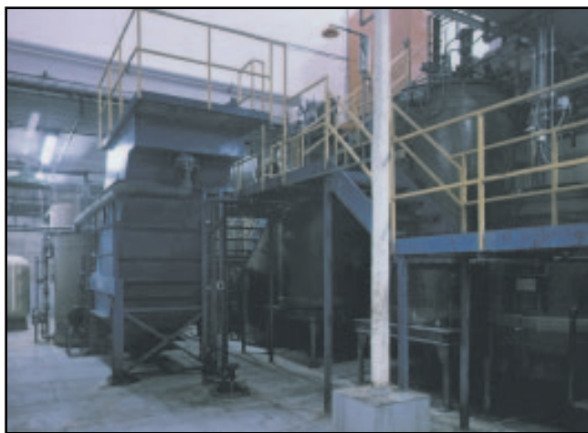
The waste treatment area is 16 ft below grade, utilizing a gravity-feed system that eliminates pumping of liquids, thereby conserving electrical energy and eliminating
