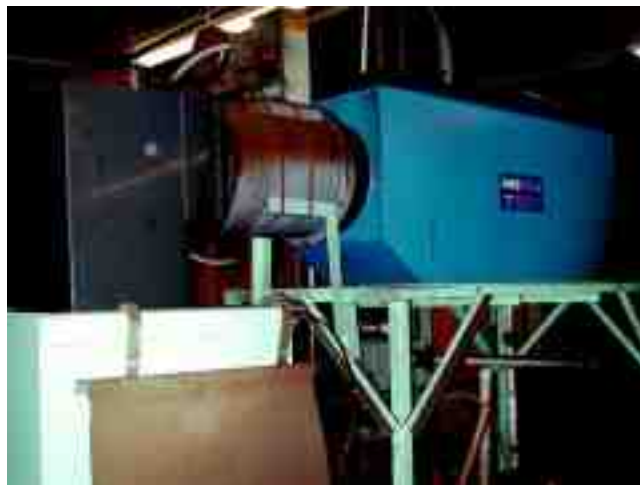
This scrubber/evaporator was modified to allow the shop to achieve zero discharge.
