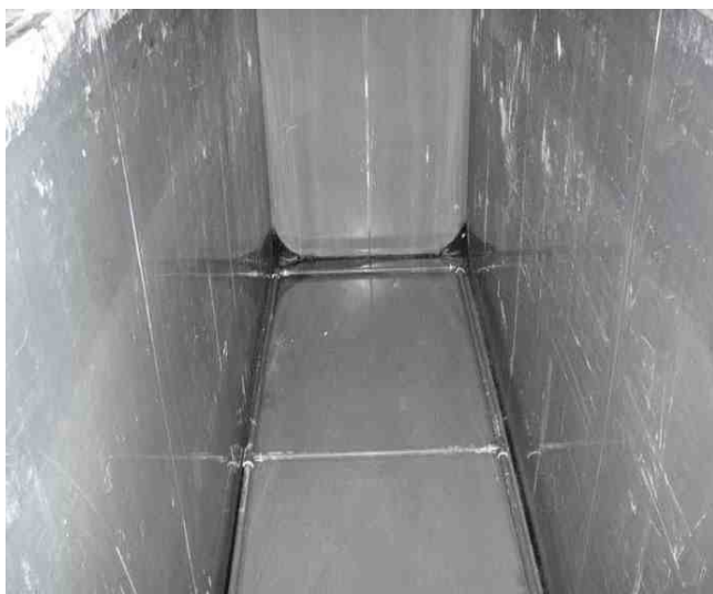
Figure 5 - Typical rigid PVC liner with extrusion welding bordering air sparger pipe, including corner inserts (patent applied for).
