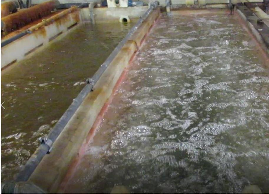
**Figure H-3. Visual Comparison of Tanks with Poor (left) and Good (right) Air Agitation**
