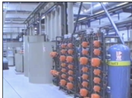
Figure 5. The wastewater treatment is carried out in batches and ion exchange of the rinse water is used to secure the quality of the final rinse water.
