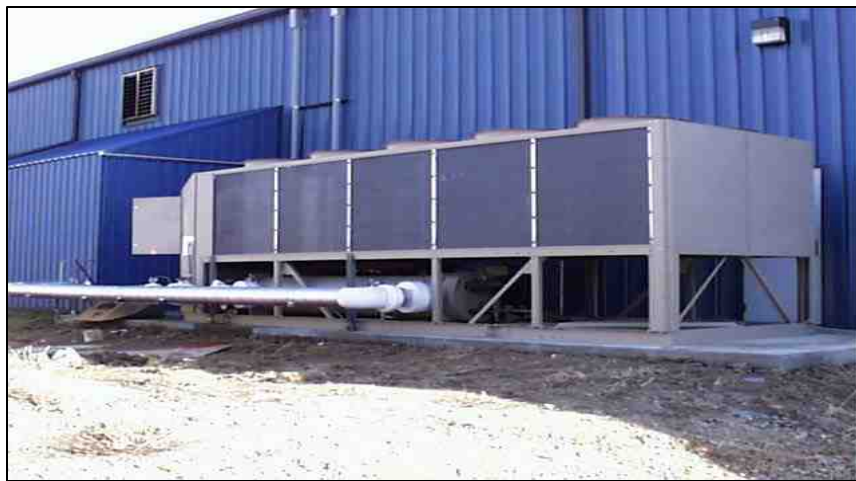
230 ton chiller installed for a hard coat type III line in Sullivan Mo.
