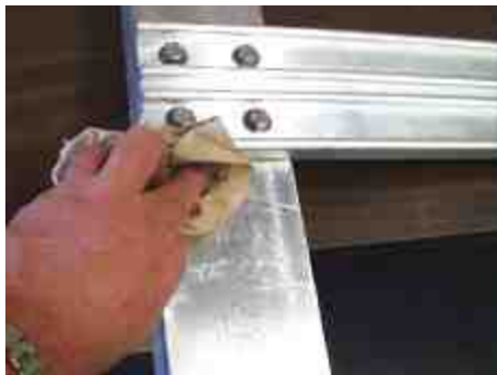
Clean excess sealant
