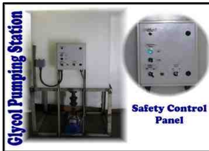
A-3 Typical glycol pumping station
