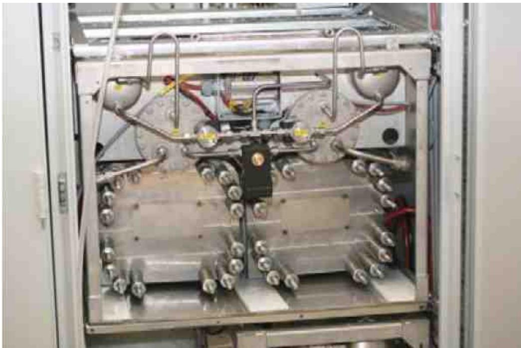
Figure 10 - Image of the electrolysis system (with two electrolysis stacks installed) produced by GreenHydrogen.dk. Courtesy of GreenHydrogen.dk.
