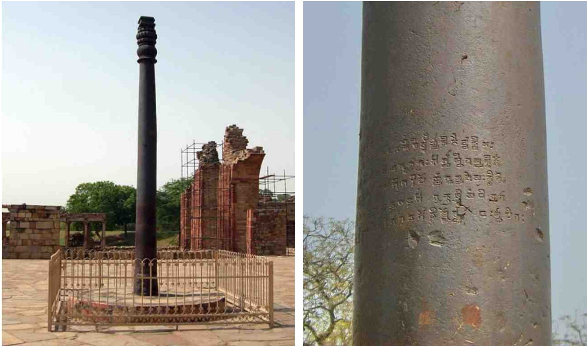
Figure 1 - (a) Iron Pillar of Delhi, 1600 years old; (b) Close-up showing minimal corrosion.
